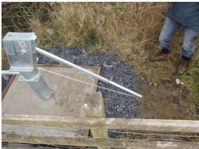
Figure 4 India Mark II handpump installed at Mount Stewart ©NERC.
