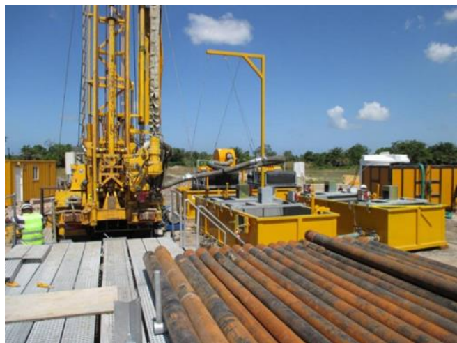
Figure 6 Reverse circulation drilling.
