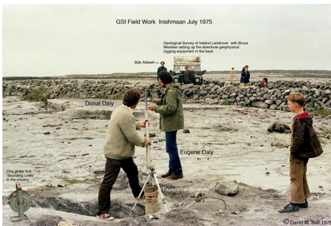
Figure 3 Setting up for geophysical logging an exploration borehole on Inishmaan in 1975. Photo by David Ball.
