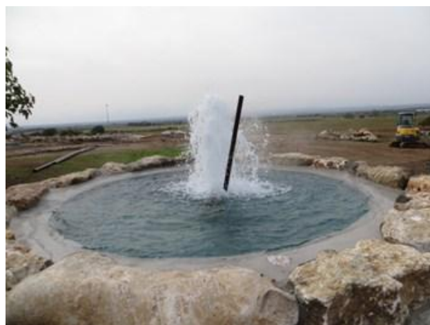
Artesian borehole discharging from volcanic aquifer
