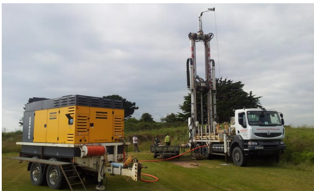
Knebel drilling rig
