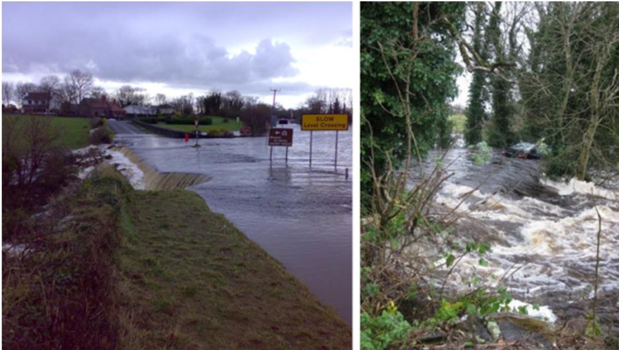
Figure 3. Flooding across the N18 National Road at Kiltartan (left) and L4506 Local Road at Corker (right) in November 2009. (Images supplied by Galway County Council)
