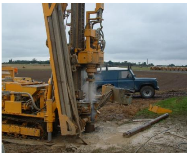
Figure 2. Drilling boreholes to investigate the groundwater denitrification capacity at a range of depths on a tillage farm
