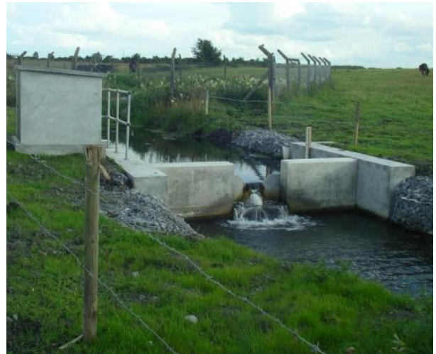
Figure 2. Weir installation at Caltra GWS, County Galway
