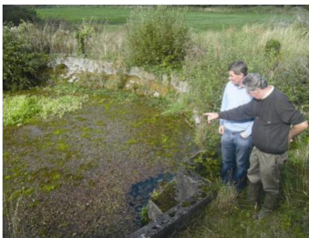
Kilriffith:Kilmore Group Water Scheme near Nenagh, Co. Tipperary. Discussion on improvements to the spring source that supplies 120 households as well as farms in the locality.
