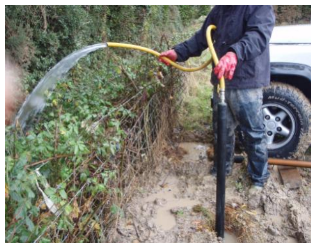
Figure 2. Confined aquifer encountered below Irish Sea till at a depth of 12m in Ballycanew. Minimum piezometric surface was 6 m above ground with a flow rate of c. 150 l/minute
