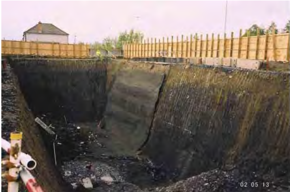
Till from the Dublin Port Tunnel excavation in Whitehall Dublin. Brown till is readily visible overlying the black till. (Photo, Eric Farrell, TCD)
