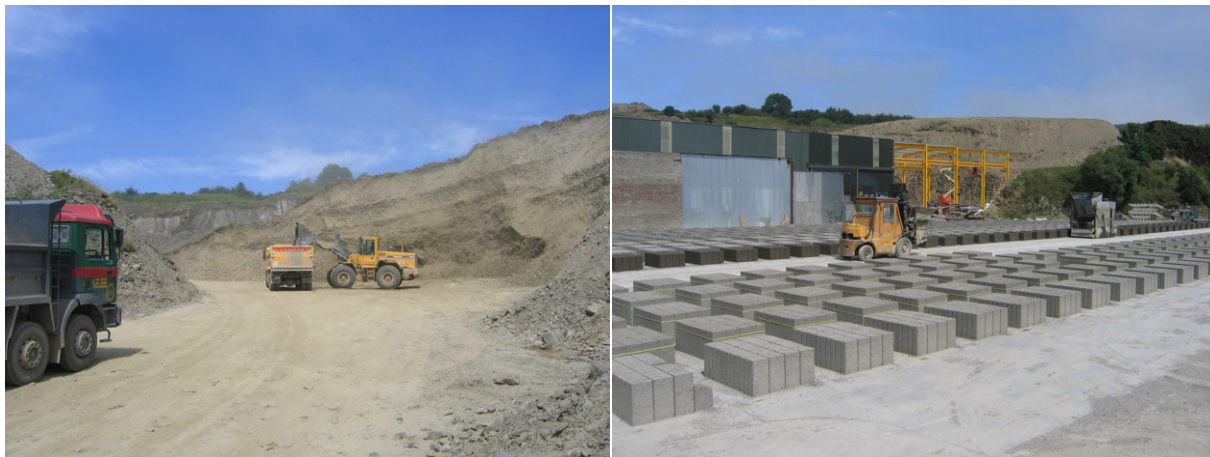
Left: Aggregate quarry within the Slate Quarries townland. Right: Concrete blocks being manufactured, made from crushed rock aggregate in Frank Murphy Ltd Slate Quarries.
