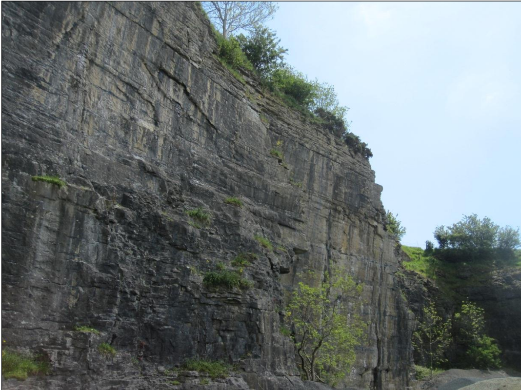
The main quarry face.
